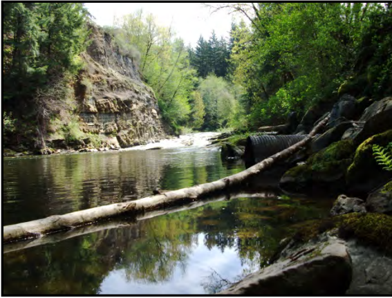
Photo 1. Upstream view of bypass chute. Note: Excavated ridge on left side of photo (August 2008).
